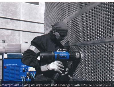
Underground welding on large-scale heat exchanger: With extreme precision and economy, the pipe welding head will produce several thousand weld seams that are as identical as two peas in a pod
